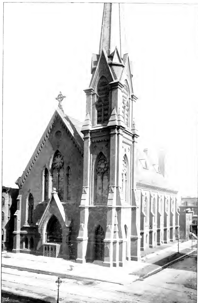
THE FIRST PRESBYTERIAN CHURCH Corner Indiana Avenue and Twenty-First Street.
